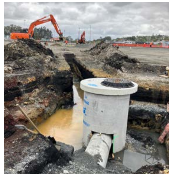
Drainage improvement work going on at the Whangārei rail yard.
