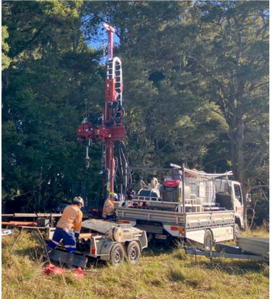
Above: core drilling near Flyers Road on the Marsden Point Rail Link route, to understand the geology. Below: ground testing at Oakleigh
