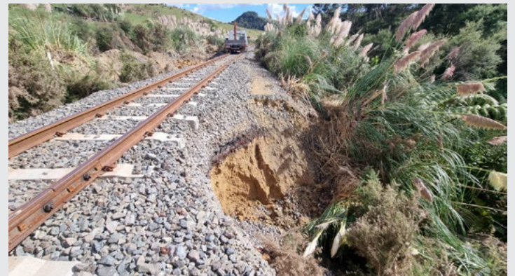
Further up the line – slips underneath the rail corridor. We will need to rebuild the hillside or put in massive retaining walls.
