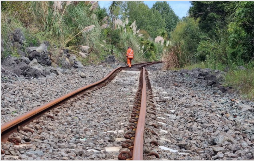
Rail line north of Tahekeroa, at the base of a large slip. We need to understand what is happening below ground.
