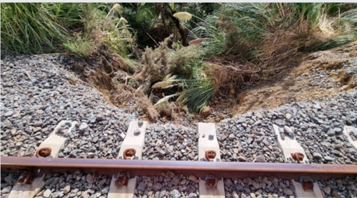
Further up the line – slips underneath the rail corridor. We will need to rebuild the hillside or put in massive retaining walls.
